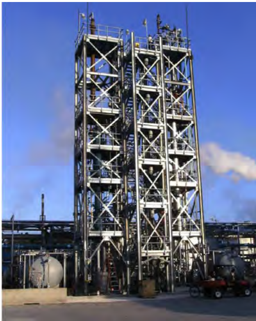
Plate 2-1: HCl Azeotrope and evaporator towers
